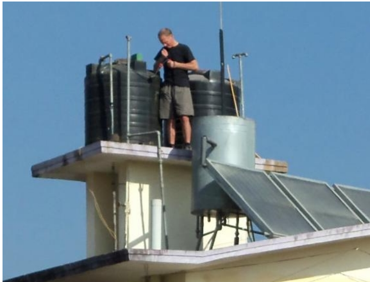
Graham up on the GSM roof checking our water system.
